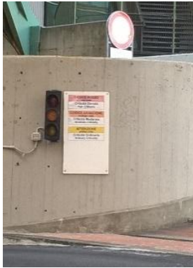
Figure 30. Warning lights in case of emergency via yellow-orange-red code 93 . (Picture by the author, May 2017)
