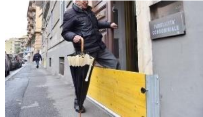
Figure 32. System of removable bulkheads for protecting shop windows and doors in case of flood. (First two pictures by the author, May 2017 94 )
