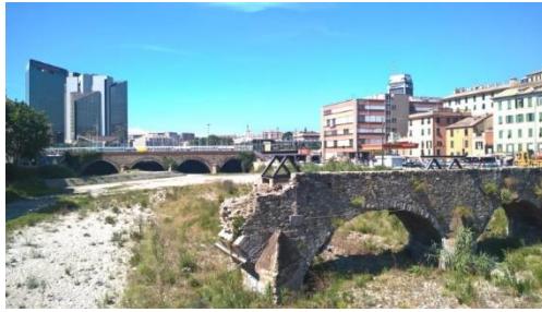
Figure 24 (a). Bisagno’s riverbed. On the background, the bridge of the railway station “Genova Brignole” (1906): the river is covered from the railway until the sea mouth. In the front, the ruins of Sant’Agata bridge (1535 92 ) progressively destroyed by 1970 and 1992 floods. (Picture by the author, May 2017)
