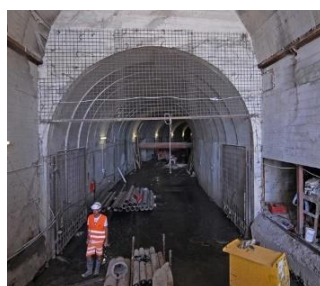
Figure 62 Internal view of the floodway 123
