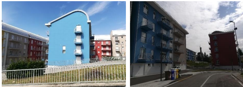
Figure 96 - Figure 97. Consorzio 201 rebuilt. Pictures by the author (September 2018)
