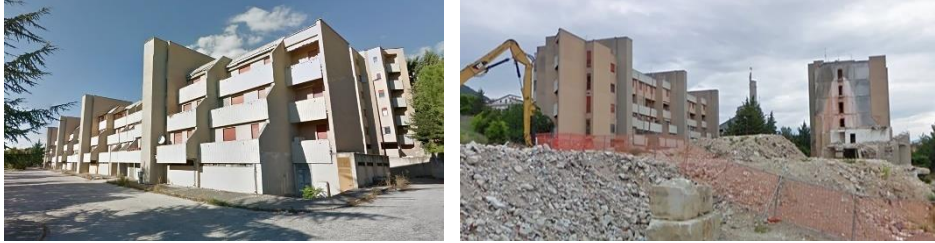
Figure 94 - Figure 95. Consorzio 201 before the earthquake and during the demolition works. (Source: Google Street View)
