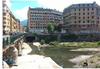
Figure 25 (b). Fereggiano’s inflow (channelled and covered) into Bisagno’s riverbed. In the right corner, a boat: they frequently reach the city from the woods through the rivers. (Picture by the author, May 2017)
