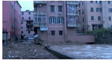
Figure 17. Building in via Giotto no. 15 during 2010 flood 82
